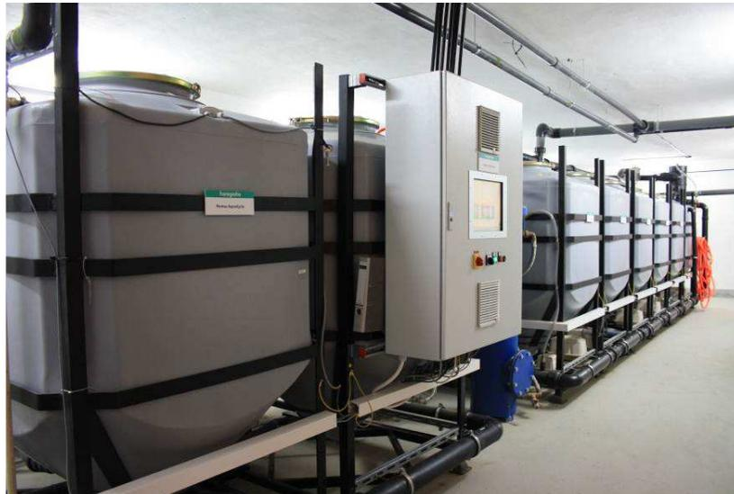
Mechanical-biological greywater treatment systems allow greywater reuse **for toilet flushing and cleaning purposes and gardening** because they are more efficient and have a UV-disinfection device. Such systems require less space and are very suitable for hotels and multipurpose buildings. More than 30 systems are already installed in the Mediterranean Area and Jordan.
